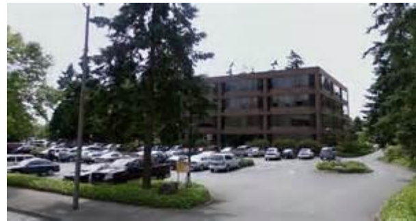
Redmond - US Development Center
